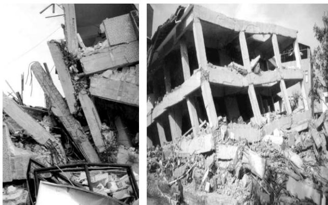
Fig. 1-1. Building structures damaged by earthquake load
