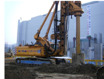
[STEP 1] Penetrating and cleaning the hole
