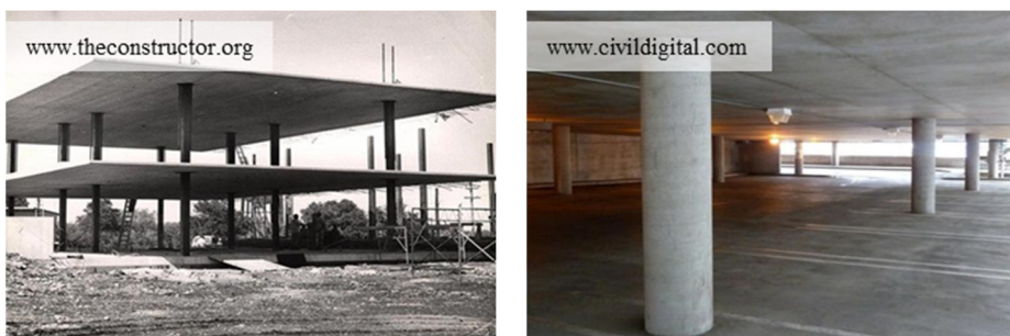
Fig 1-1. Flat plate system
