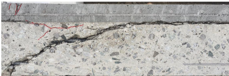
(b) Inclined shear, flexural and near interface crack in specimens
