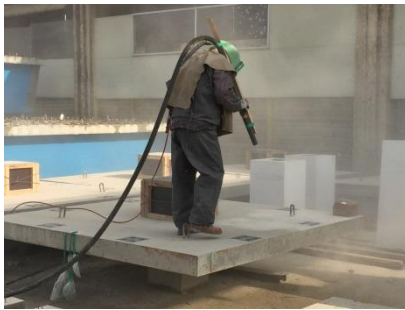
(a) Interface sand-blasting
