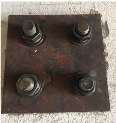
(b) Steel plate anchored at supports
