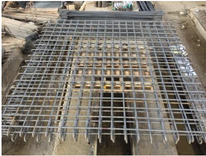
(a) Arrangement rebar
