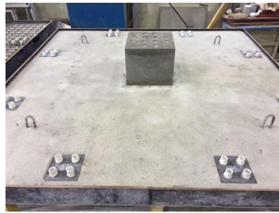
(b) Formwork installation
