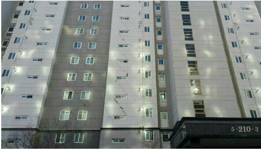
Figure 1-2 Damage of the Pohang earthquake
