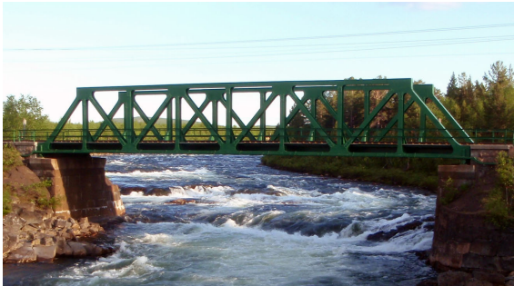
Figure 1: A photo of the Rautasjokk Bridge
