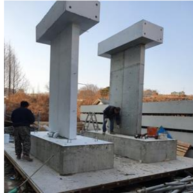
(f) Completed specimen.
