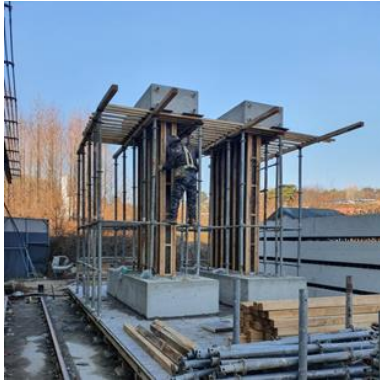
(g) Concrete pouring into head beam and curing
