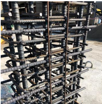
(a) Assembly of U-tie module
