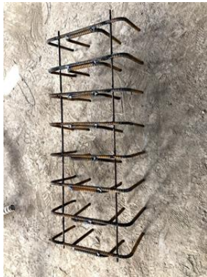
(c) Fabrication and assembly of transverse details
