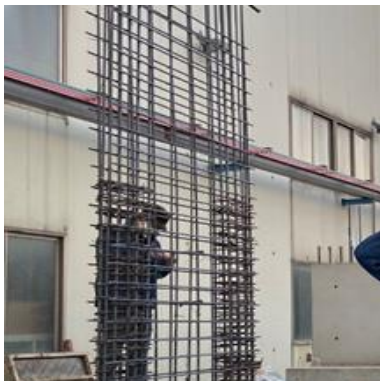
(e) Attaching the strain gauge
