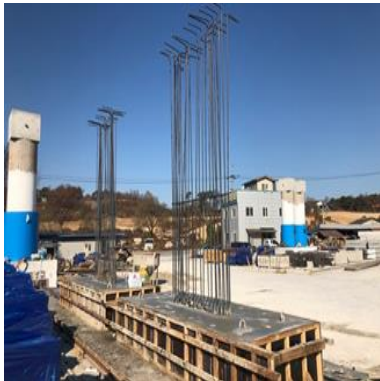
(c) Foundation concrete pouring and curing
