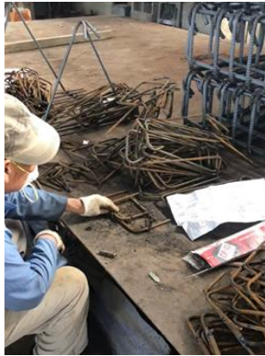
(a) Rebar processing
