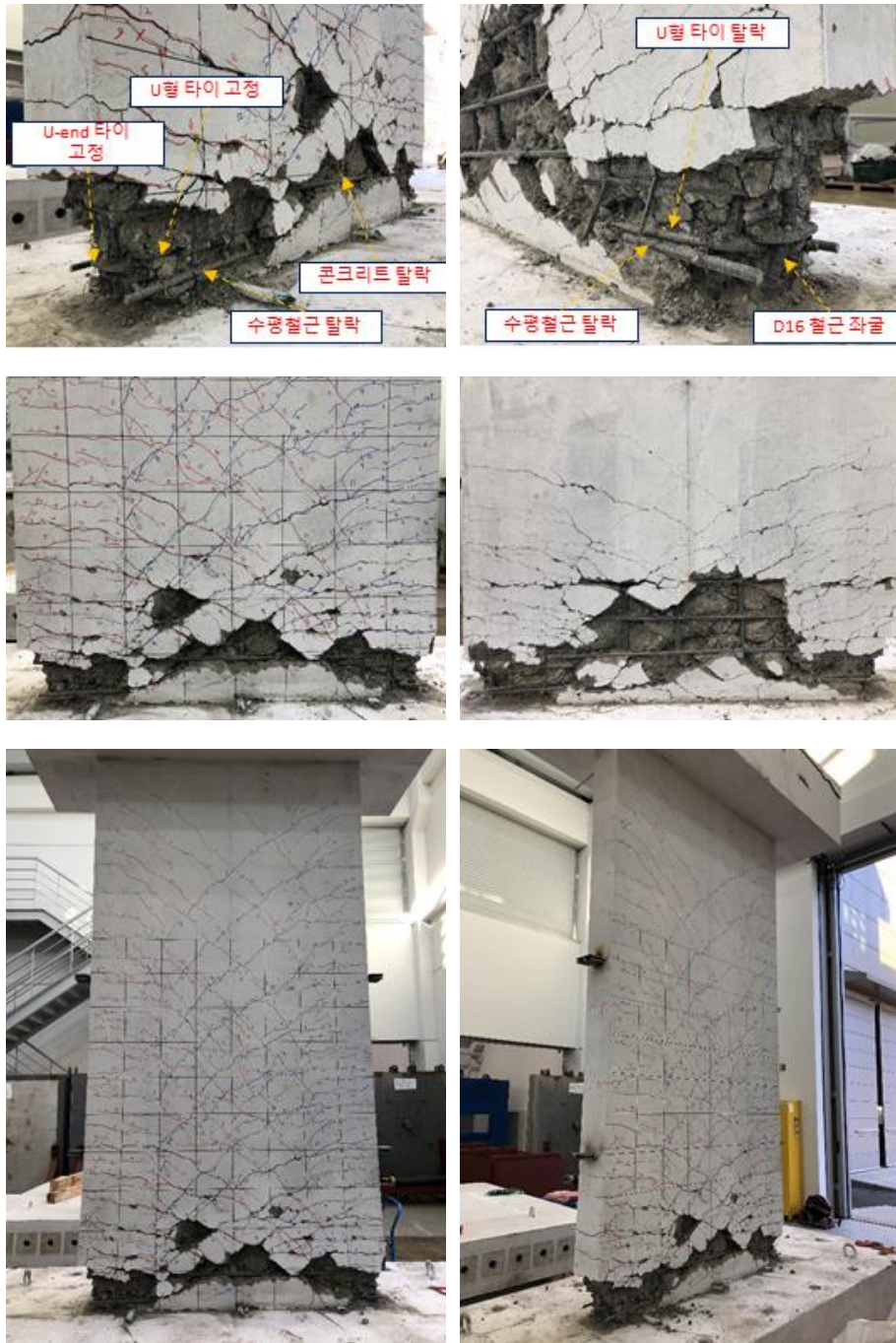
Figure 4-10 Crack and failure mode of WS2
