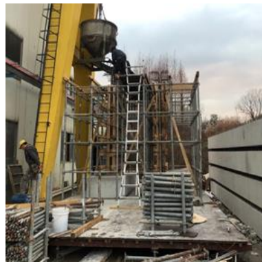
(f) Concrete pouring into wall and curing
