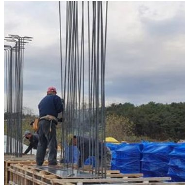
(b) Assembling the rebar for foundation, head beam, wall
