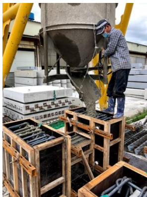
(e) Concrete pouring and curing
