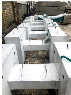
(f) Completed specimen
