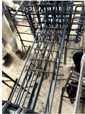
(b) Assembling the rebar for foundation, head and boundary element
