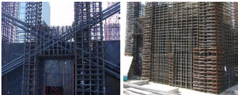
Figure 1-3 Details of reinforced concrete shear wall
