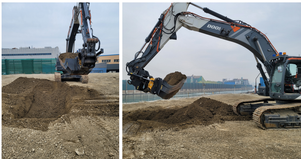
FIGURE 4.1: Experiment environment using tilt-rotator excavator
