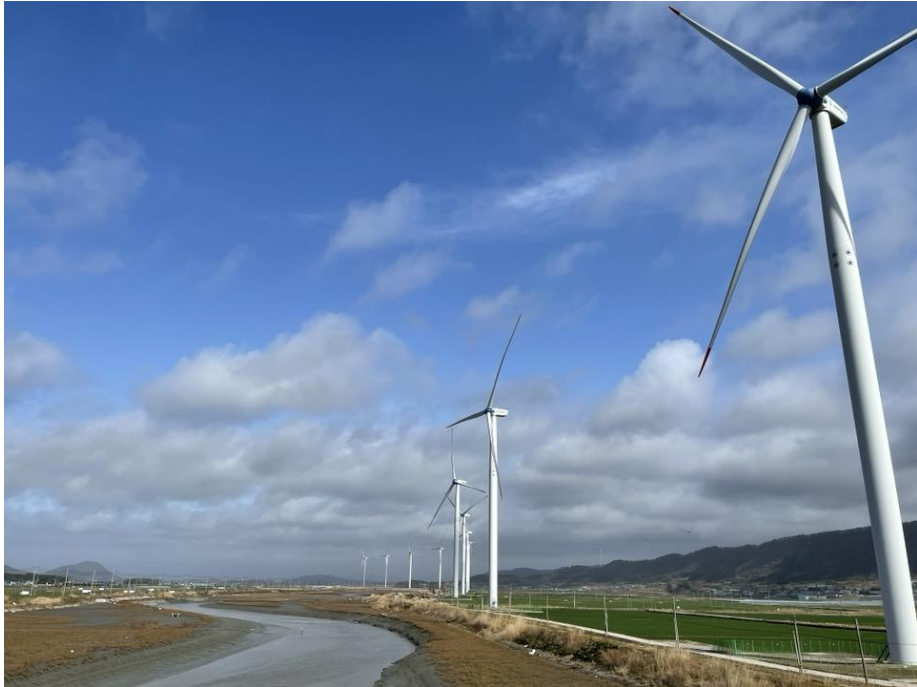
Figure 2. Wind turbines in the study area
