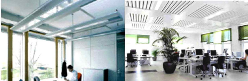
(a) passive chilled beam
