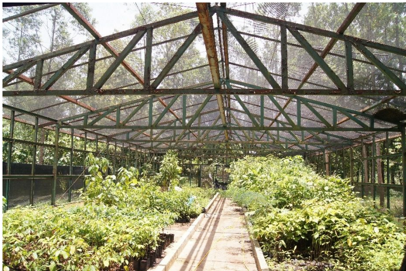
Figure 1 The view of the open nursery with sun screen at the top
