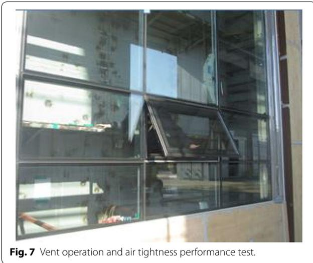
**Fig. 7** Vent operation and air tightness performance test.
