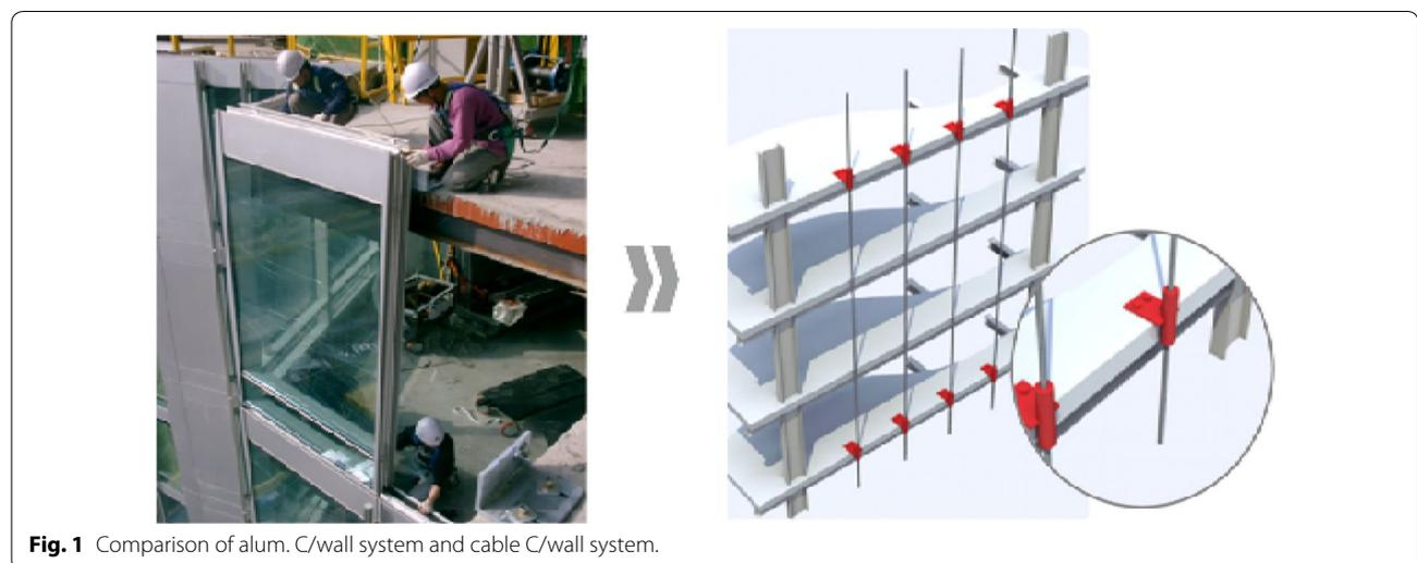
**Fig. 1** Comparison of alum. C/wall system and cable C/wall system.
