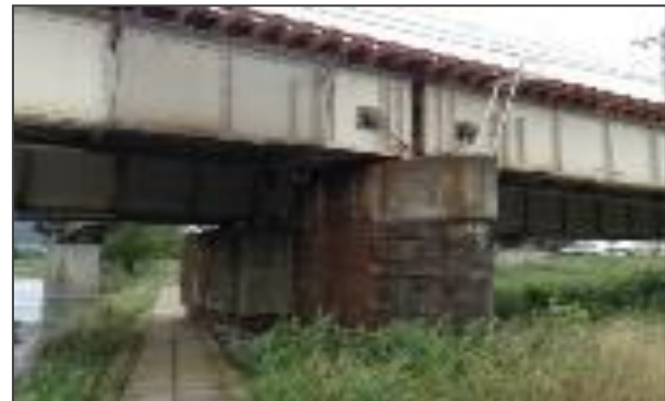
(a) Before repair
