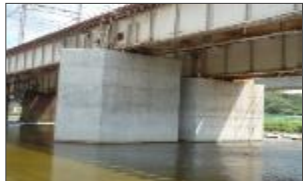
(b) After reinforcement
