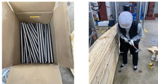
Figure 5-3 Titanium bar and inserting process
