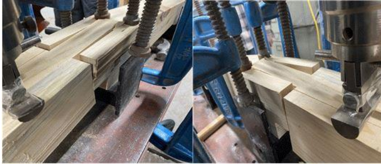
Figure Appendix.B. 21 Repaired 2 of Mok-gi-yeon
