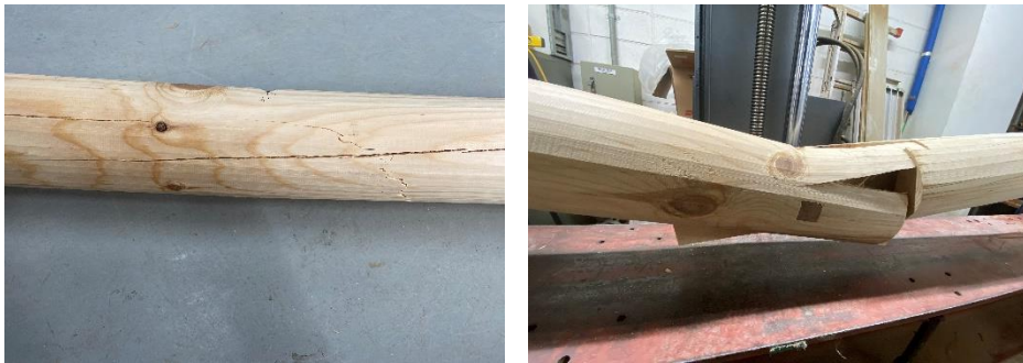
Figure Appendix.B. 6 Reference 3 (left), Repaired 1(right) of Jang-yeon
