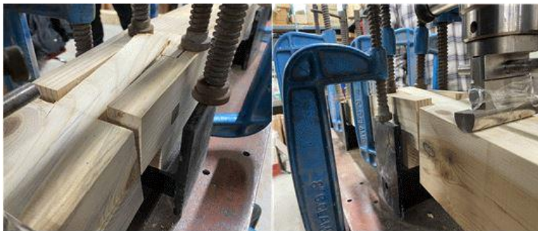
Figure Appendix.B. 22 Repaired 3 of Mok-gi-yeon
