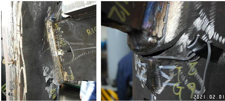
(b) Chord punching shear failure
