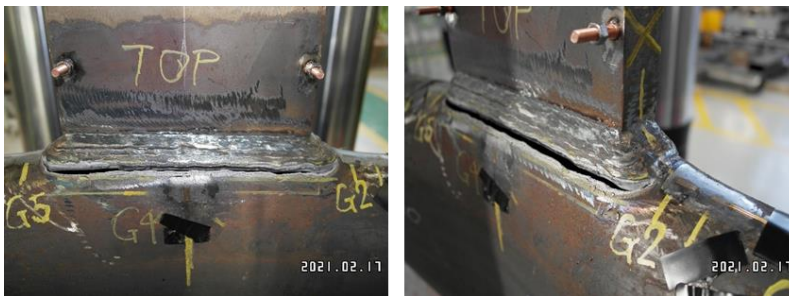
(b) Chord punching shear failure
