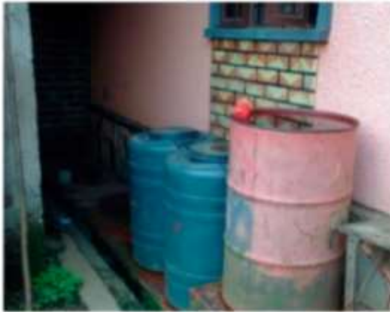
Figure 2. Informal steel barrel rainwater in Uganda (Kisakye, Akurut and Van der Bruggen, 2018)
