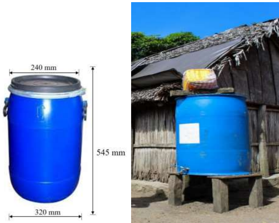
Figure 4. Dimension of plastic drum of 30 L and a roof rainwater harvesting system with a plastic drum in Madagascar (SEED Madagascar).
