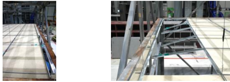
(b) Perimeter ceiling panel displacement
