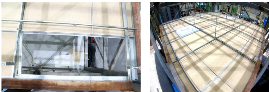
(b) Damage observed at the end of test
