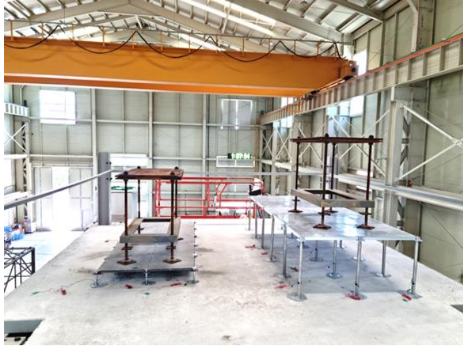
Figure 4.5 FH150-S and FH300-S specimens installed on the roof of 2-story steel frame
