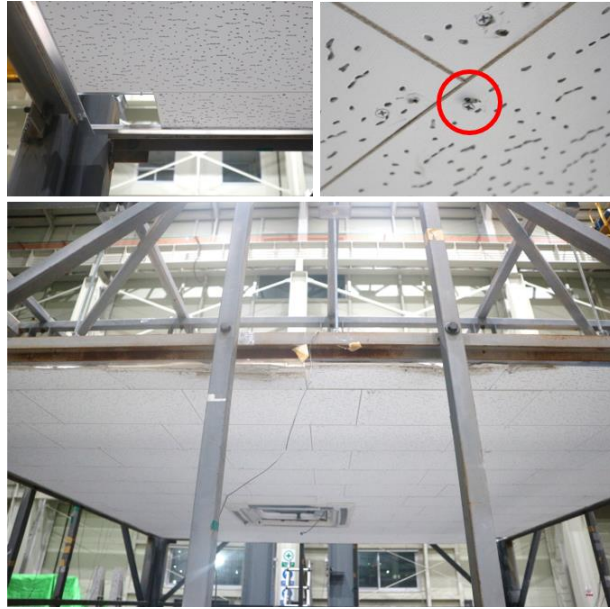
Figure 5.25 Failure pattern of IMC specimen observed during shake table test
