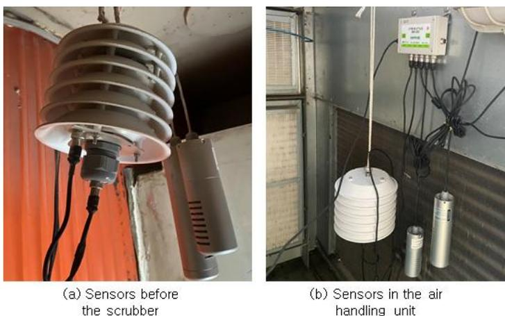
**Figure 18** Installed sensors with sensor node
