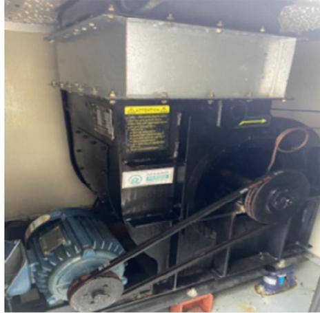
**Figure 9** Fan in air handling unit
