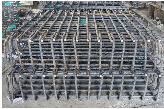
(a) assembly of reinforcement
