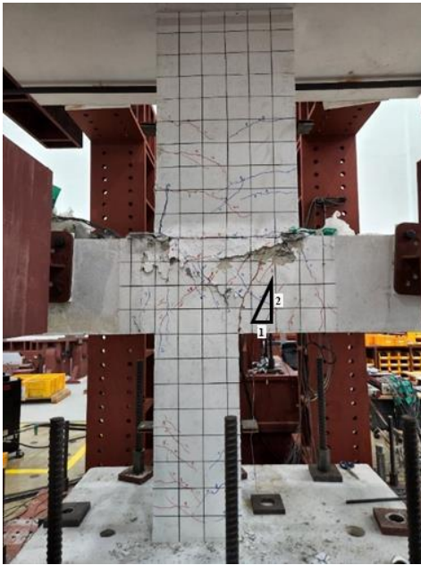
(a) Crack of vertical member
