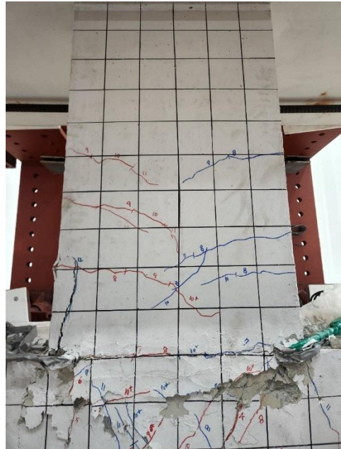
(b) Flexural failure of wall
