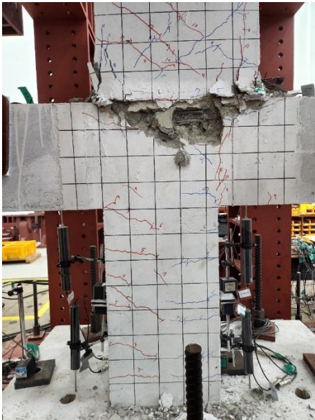
(a) Crack of vertical member
