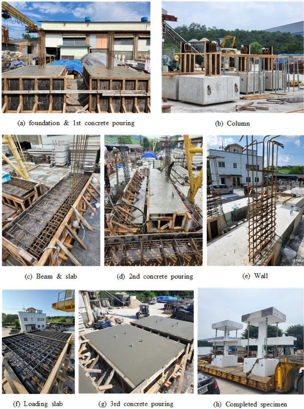
Figure 4-18 Construction procedures of the specimens
