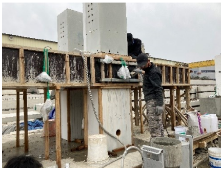
(c) Injecting non-shrinkage grout
