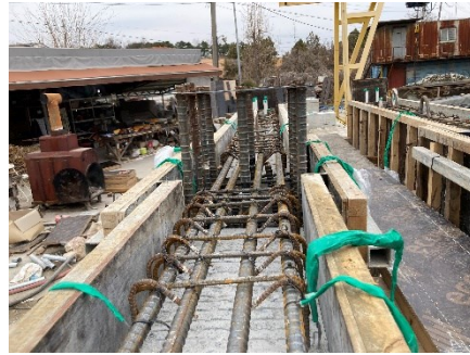
(b) Assembling beam top bars and stirrups
