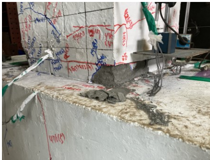
(a) Grout cover delamination ( \delta = 1.5\% )
