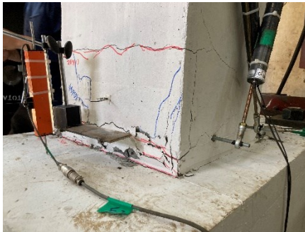
(a) Concrete cover cracking ( \delta = 2.0\% )
