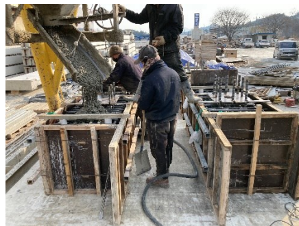
(b) Placing concrete
