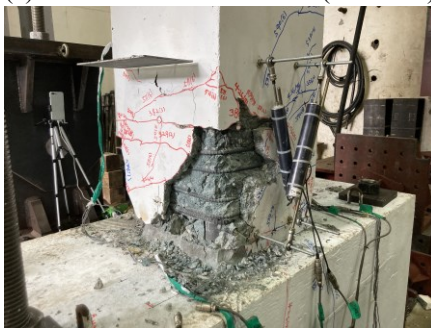
(c) Sleeve cover spalling of a tensile side ( \delta = 4.5\% )
