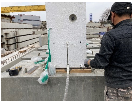
(c) Injecting non-shrinkage grout
