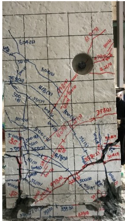
(e) Final failure (front) ( \delta = 3.5\% )
