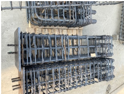
(a) Assembling steel cages
