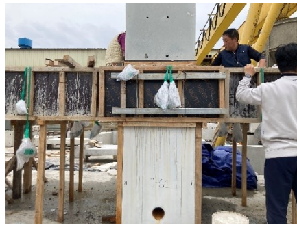
(b) Assembling upper column and manufacturing mold
