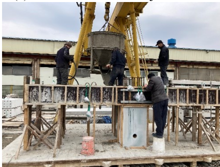
(e) CIP topping and joint
