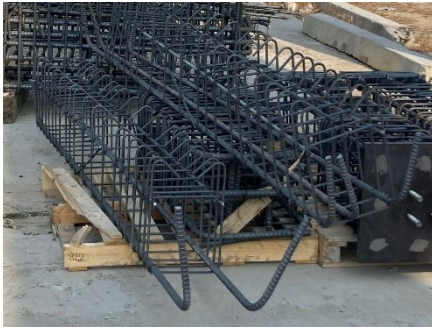
(a) Assembling steel cages
