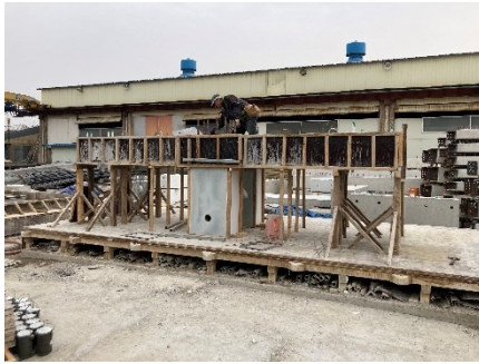
(a) Assembling members and manufacturing mold
