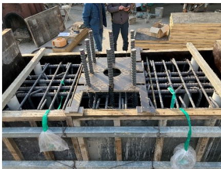
(a) Assembling steel cages · Attaching strain gauges · Manufacturing mold
