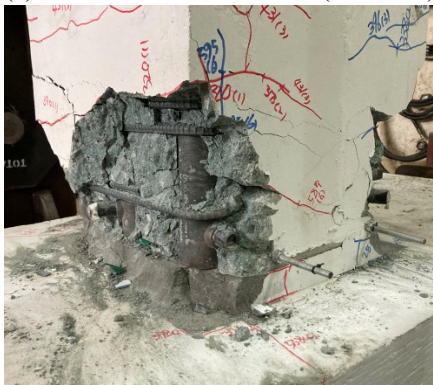
(c) Sleeve cover spalling of a tensile side ( \delta = 2.75\% )
