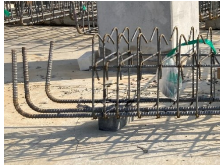
(b) Attaching strain gauges
