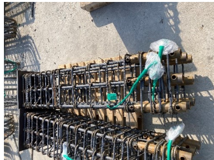
(b) Attaching strain gauges
