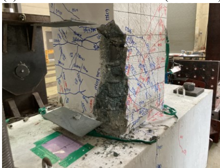
(c) Sleeve cover spalling of a tensile side ( \delta = 2.0\% )
