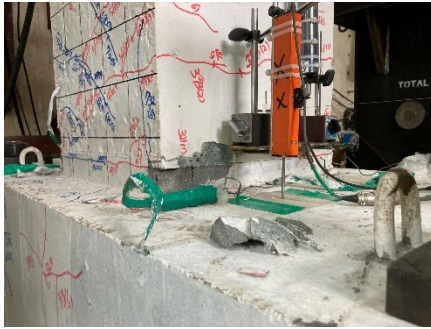
(a) Grout cover delamination ( \delta = 1.5\% )
