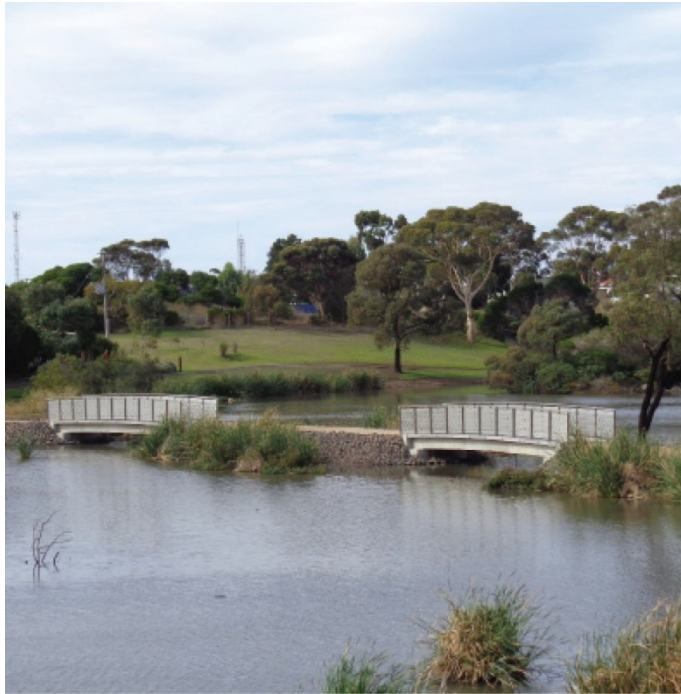
Figure 2-11 Geopolymer concrete footbridge
