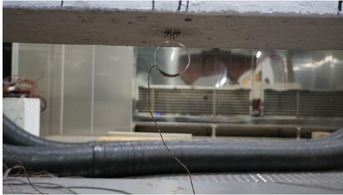
Figure 3.24 Crack gauge at bottom of RC beam
