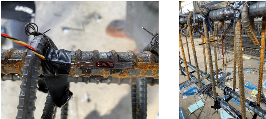
Figure 3.7 Installation of strain gauges and thermocouple
