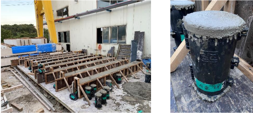
Figure 3.9 Fabrication of RC beams and concrete cylinders
