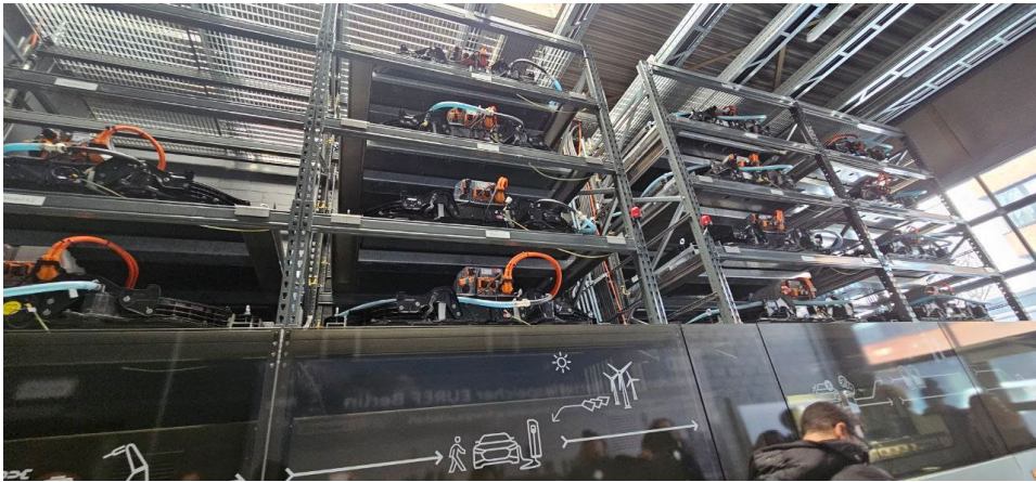
Figure 4.3 Reused battery from EV as UBESS in EUREF Campus Berlin
