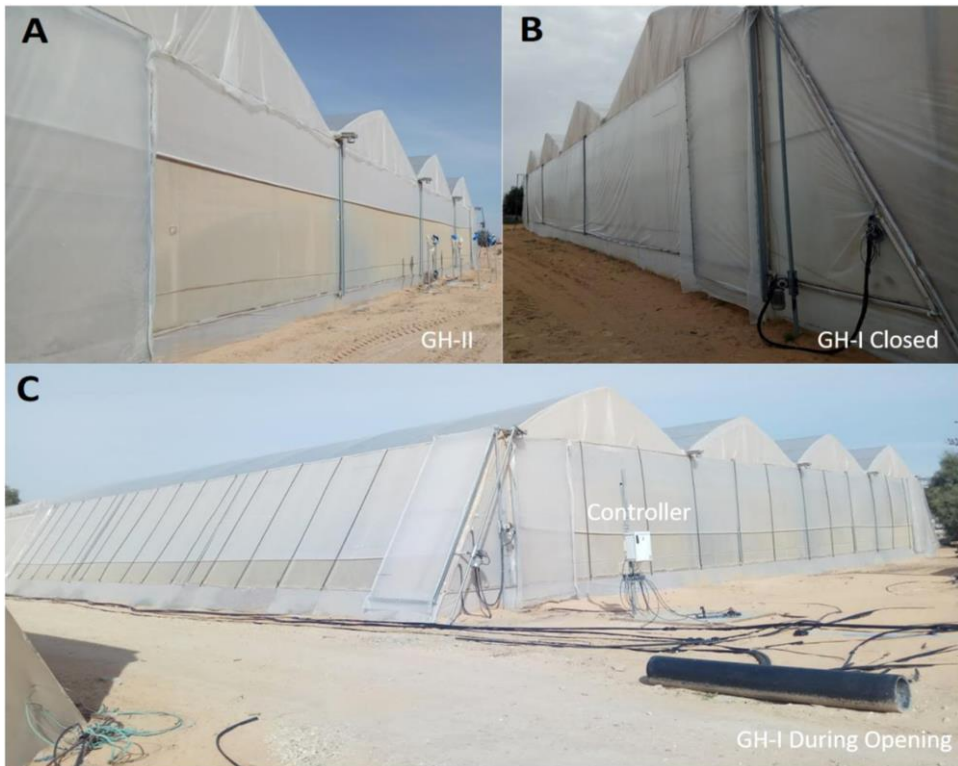
Figure 2-2 Outside view of the naturally ventilated greenhouse(GH-II) at the north position(a), lateral controller, and curtains closed in the semi-closed greenhouse(GH-I) at the south position (B). General view of the semi-closed greenhouse(GH-I) during an opening event(C) (Saadon et al., 2014)
