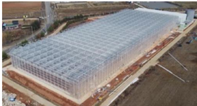
Figure 2-1 Foreground of Venlo-type advanced digital greenhouse with high elevation (Lee et al., 2022)
