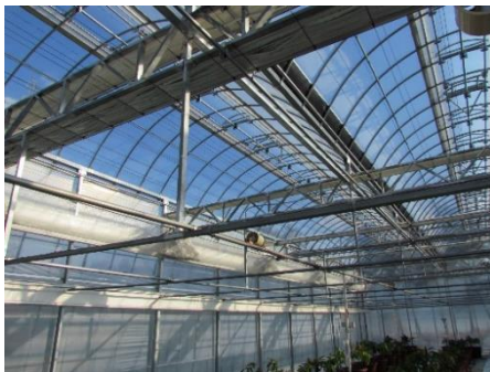
(c) roof vent opening
