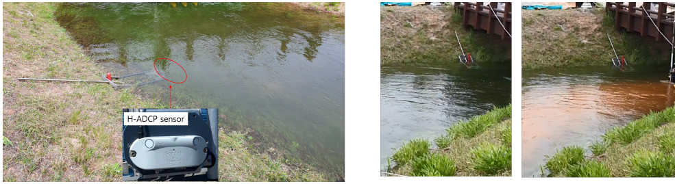
Figure 7.6 H-ADCP installation at a bank with sediment cloud passing
